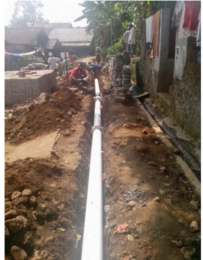
Construction of the “Eco-drain” in Bogor
