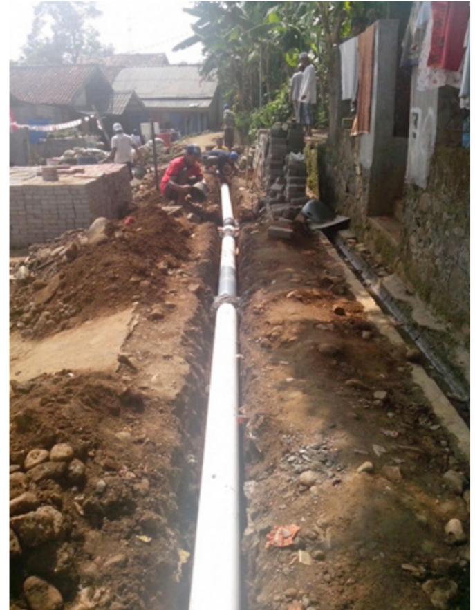
Construction of the “Eco-drain” in Bogor
