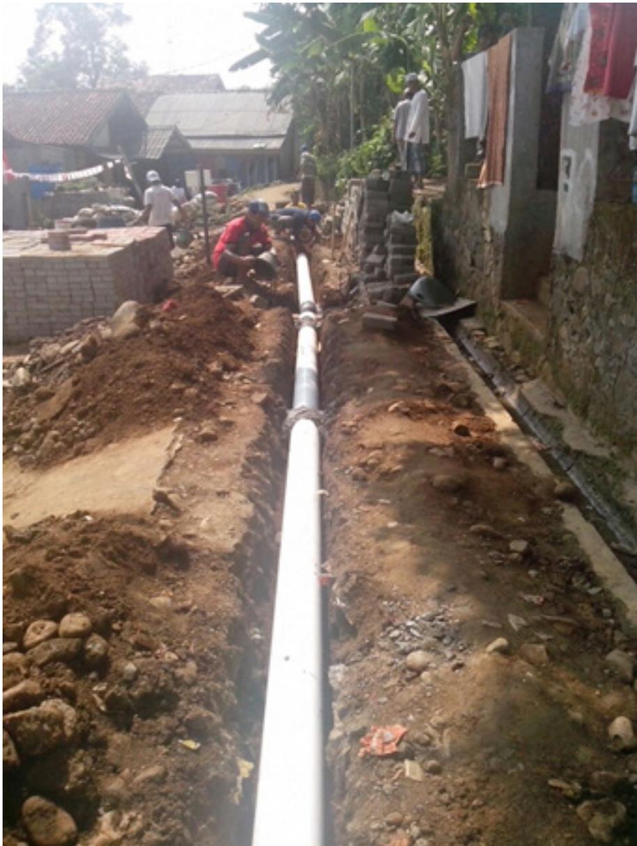
Figure 2: Construction of the “Eco-drain”
